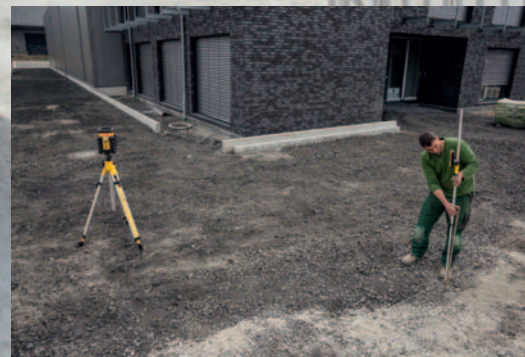
Application example: Levelling paving with up to 5° inclination.
